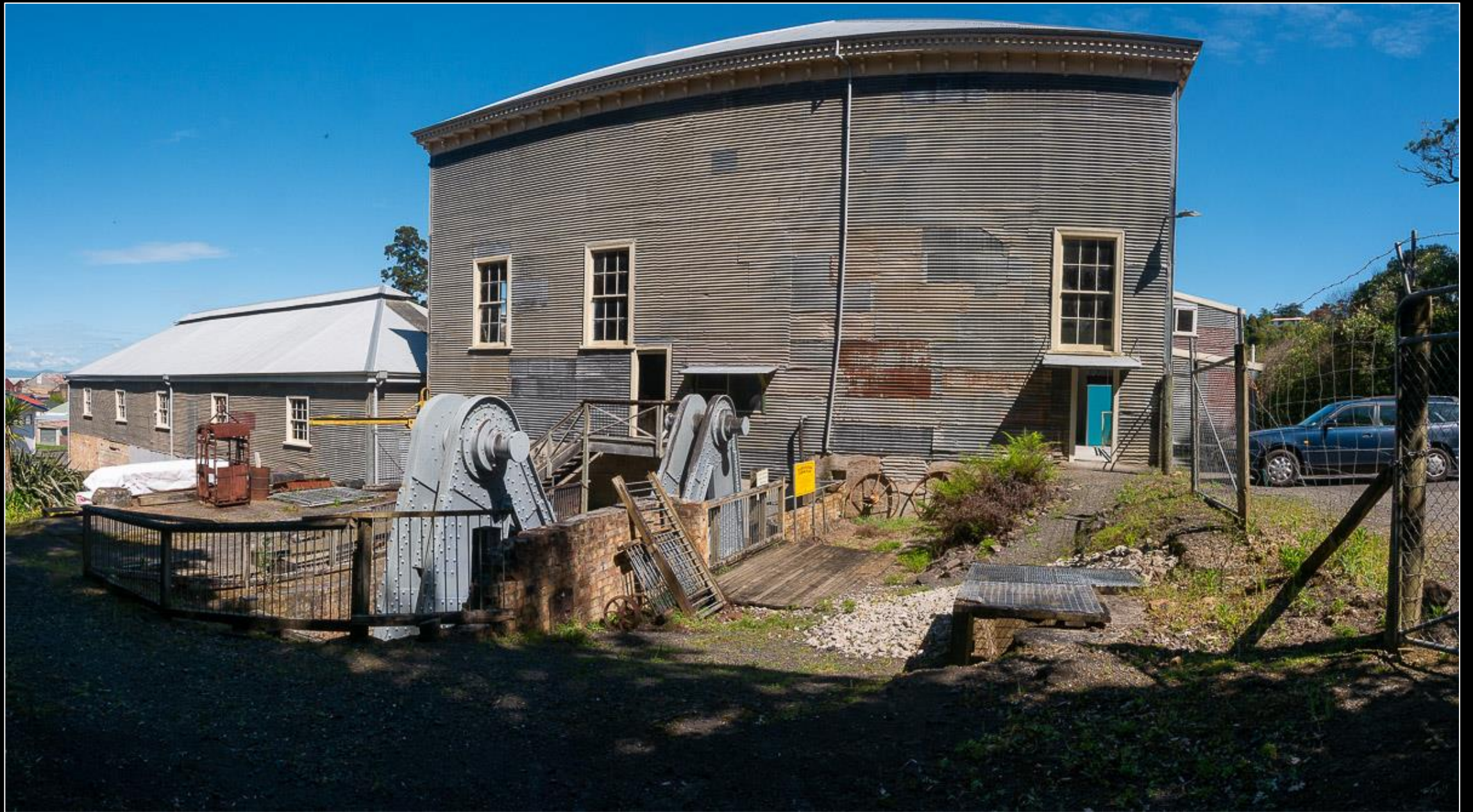
Thames Hauraki Pumping Plant 1898-1914
