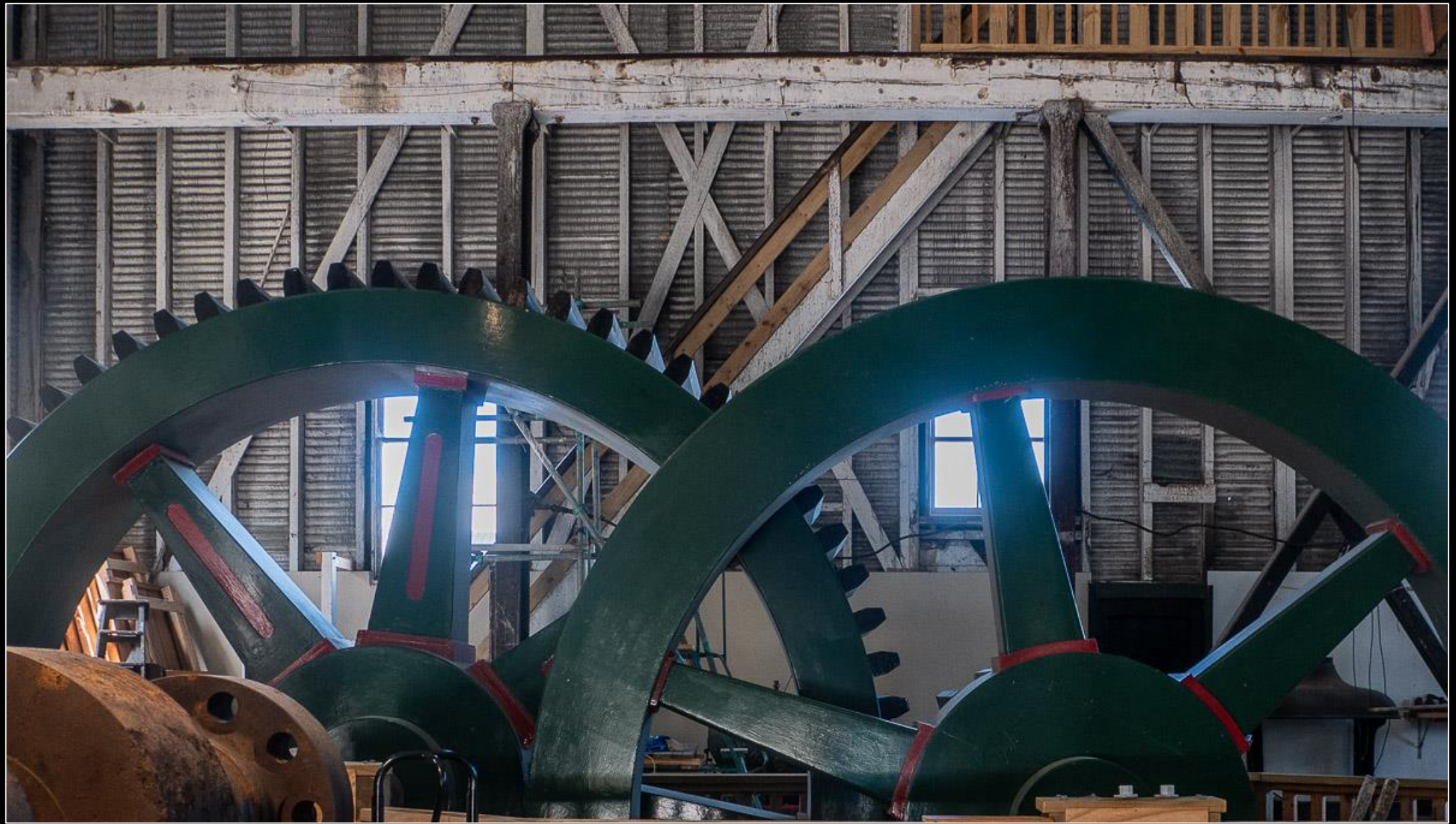
Thames Hauraki Pumping Plant 1898-1914
